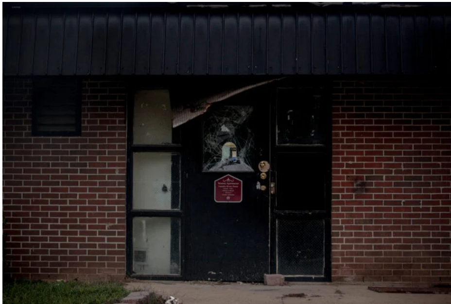
The office building at the now-shuttered Warren Apartments, which was owned by Global Ministries Foundation. (Andrea Morales, special to ProPublica)
